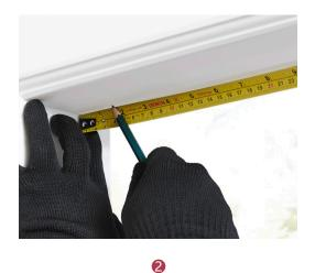
Write down the groove measurements. Put the measuring tape inside the window frame and mark where the grooves will go. Make sure the markings are lined up.
